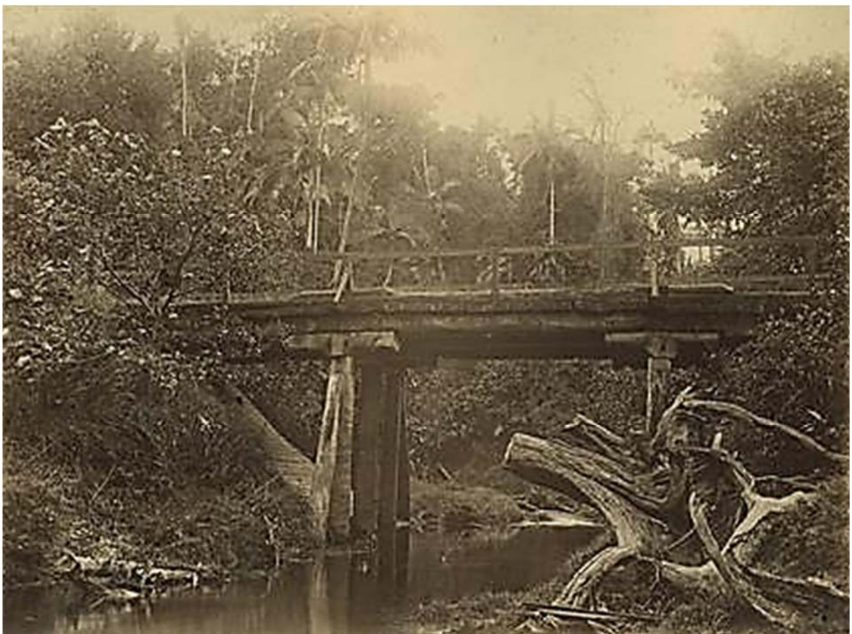
Timber Bridge over Ripple Creek
