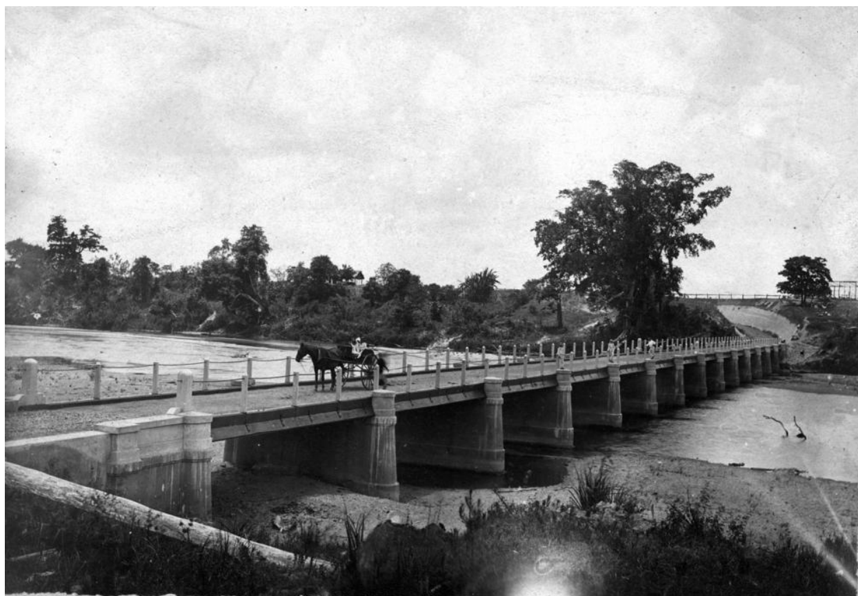
Gairloch Bridge over the Herbert River, ca 1892. Looking south
