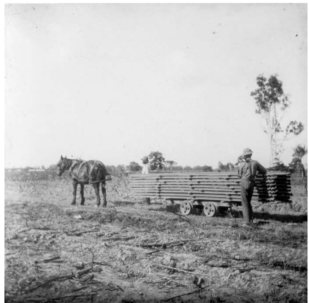
Laying horse-drawn tramway
